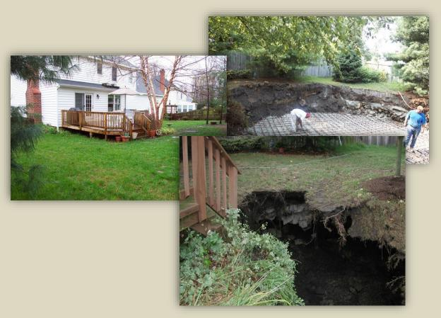
A vertical opening was discovered by DMLR during the inventory process. The property owners were contacted and informed of the AML feature on their property and agreed to have it reclaimed. The vertical opening was filled and capped, and typical marker posts were installed to indicate its location.
