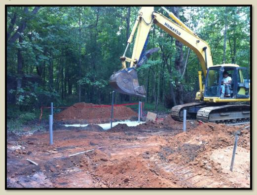
The contractor is re-grading the reclaimed shaft to the approximate original contour of the land before mining. The area will then be seeded for re-vegetation. Metal posts demarcate the location of the reclaimed shaft.
